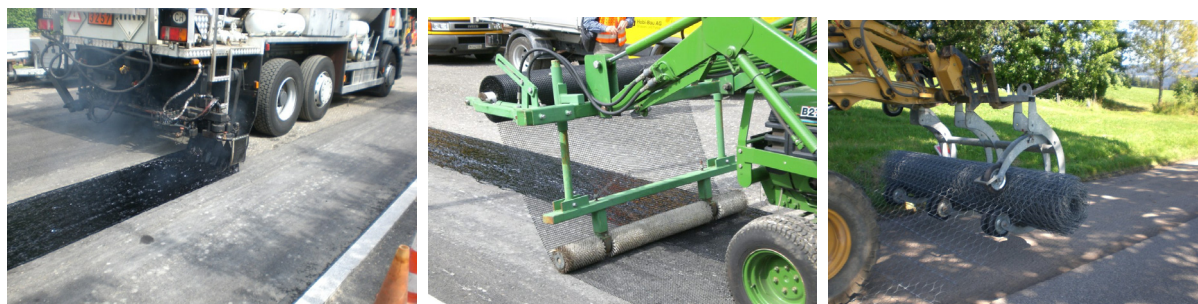
Figure 9 Installation of asphalt interlayers
